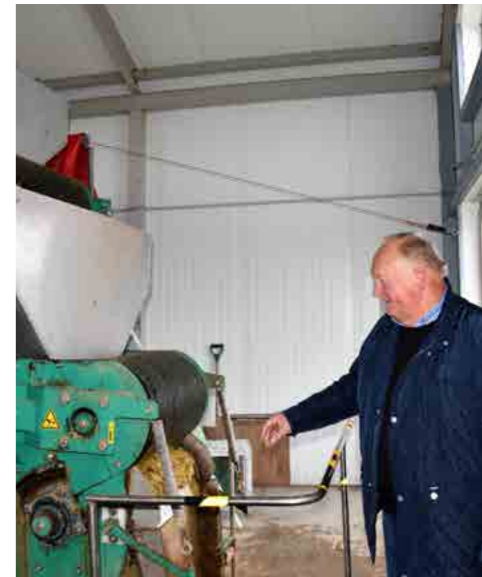
One of the state-of-the art separation systems in the Baltic States
